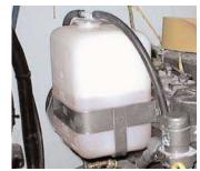
If coolant is draining down frequently, engine or generator may have a leak that needs to be serviced. Inadequate engine coolant can cause severe engine/generator damage.
